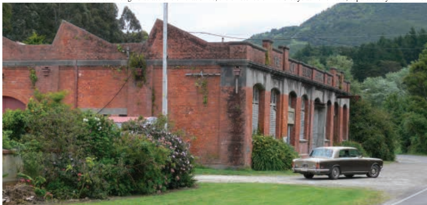
SBH10636 beside the remains of the New Zealand Shipping Company’s wool-store at Tokomaru Bay, a relic of an era when international cargo ships used the port, up until the 1950s.
