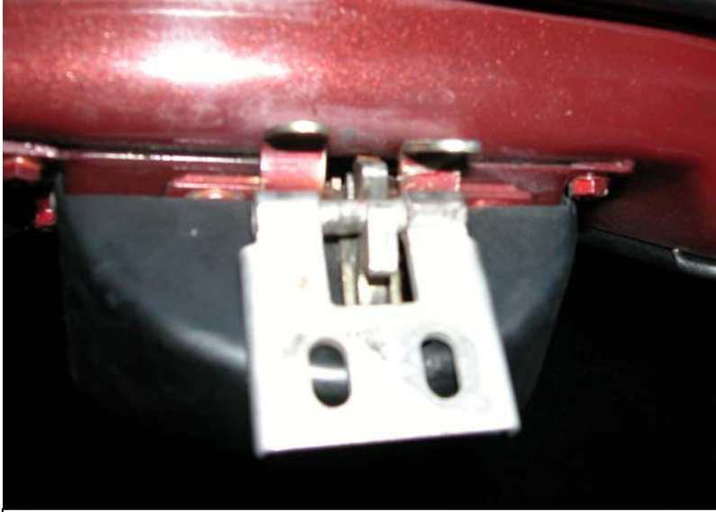
This was the welcome sight I got when the last bolt was undone. This technique I think would work on the very much later cars as they fiddled with the spare wheel stowage.
